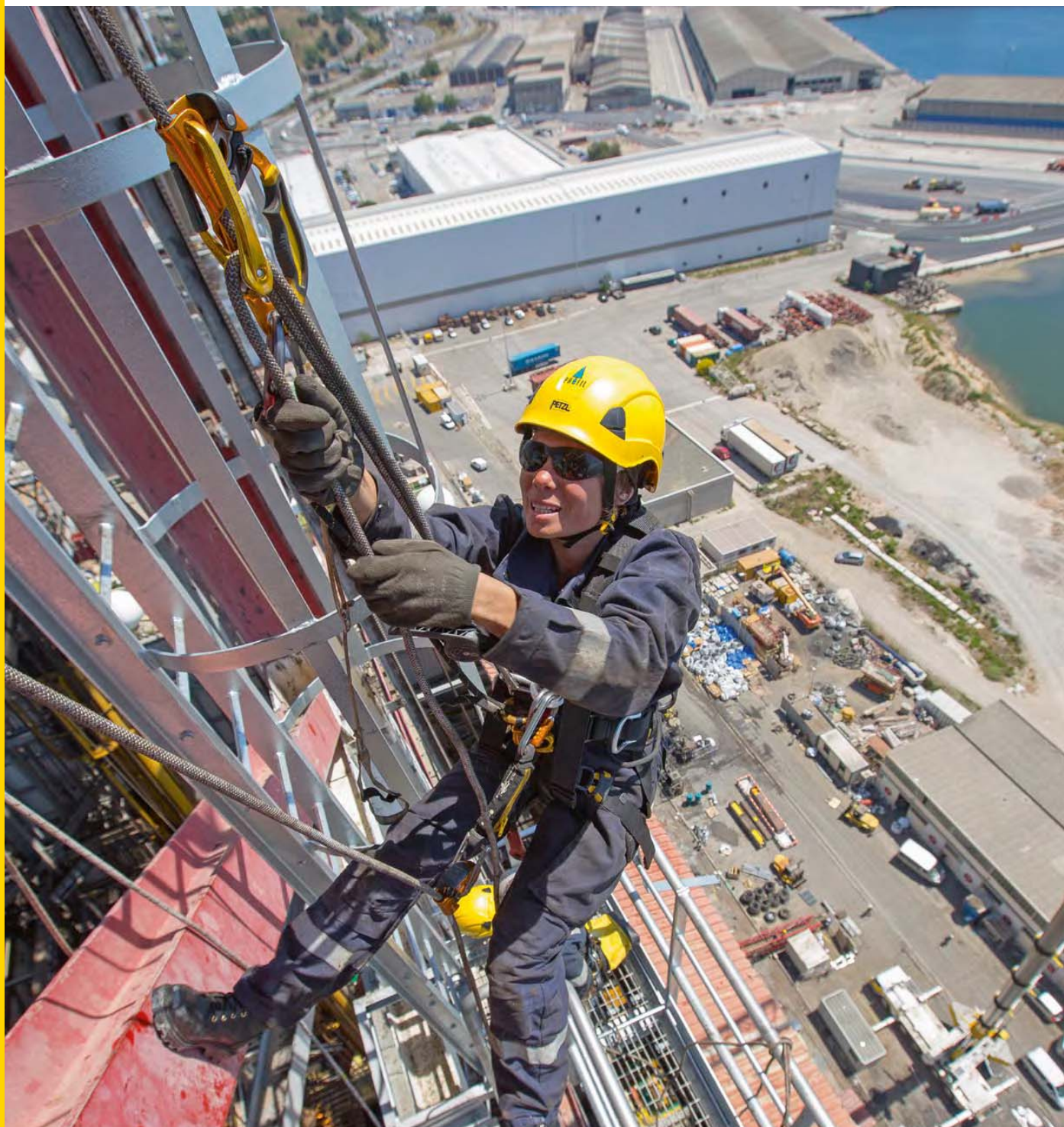
Attaching caged ladders to a derrick boat. © vuedici.org / Profili Energy
